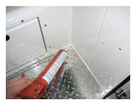
Silicone all seems and joints. This will allow the unit to be hosed out.
